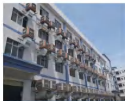
日用品车间 Daily Necessities Workshop
