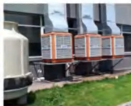
五金厂 Hardware Factory
